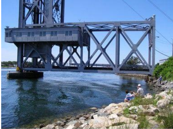
Cut: Cape Canal RR Bridge Caption: Location of where the BBTS will be installed by the end of 2016
